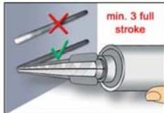
5. Prior to dispensing into the anchor hole, squeeze out separately a minimum of three full strokes and discard non-uniformly mixed adhesive components until the mortar shows a consistent grey or red colour.
